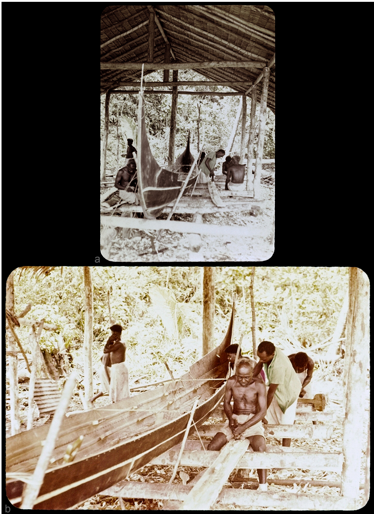
Figure 7. (a) Canoe construction at Moli, Choiseul in 1958. (b) Sewn canoe at prow, Choiseul. Photo Harold Scheffler 1959. Harold Scheffler Papers, MSS 481. With the courtesy of © Jan Simpson and Special Collections & Archives, University of California, San Diego.
