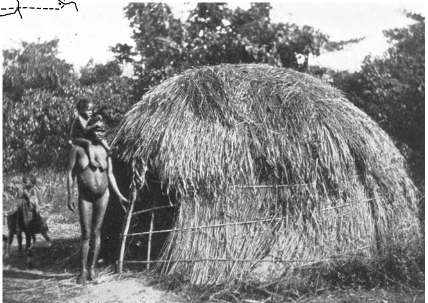
[RIGHT] Completed hut, thatched with “blady-grass” over a wityh frame-work of hoops. Lower Tully River. Roth, W.E., 1910. Bulletin 16, pl.xii, fig. 2.
