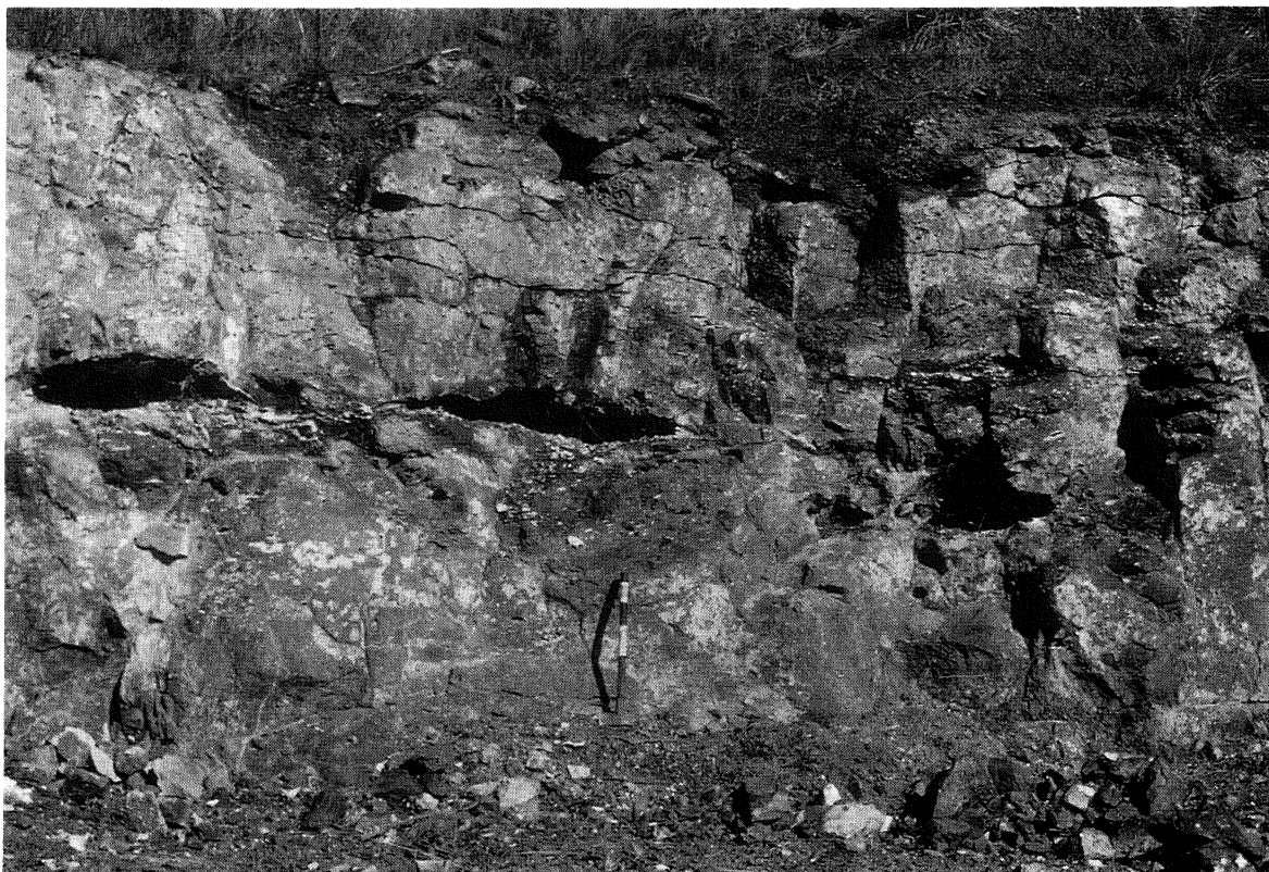
Fig.2. Large lensoidal cavities exposed in the quarry face. Depth of section is approximately 3 m. Photograph by the author.
